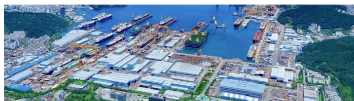
The Hanwha shipyard, Port of Okpo, South Gyeongsang Province, ROK.
